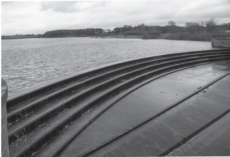
reservoir overflow steps
